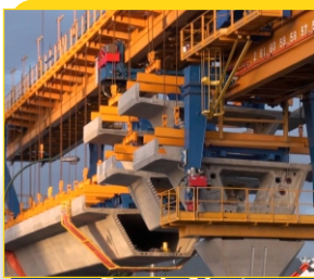
Fund, Abuja Construction- Road/Bridges
